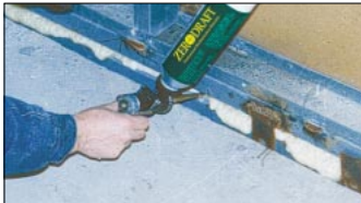
Zerodraft Foam Sealant being applied to base of wall.
