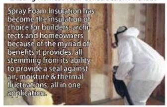
Closed-Cell Spray Foam Insulation outperforms traditional insulation by providing an air, water & vapor barrier in a single component.
